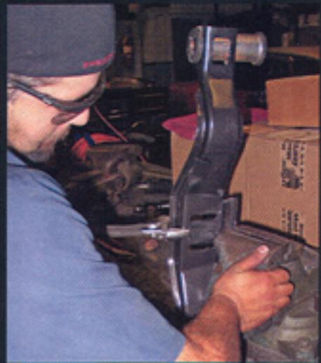
▲ The factory crossmember requires an extensive amount of modifying to get it to work with the AODE's longer tail section. In this photo, Saul uses a vise to straighten out a flat-like extension plate cut from the original crossmember. He then welds gussets to each end that triangulate and strengthen the plate, and readies it for supporting the transmission.
